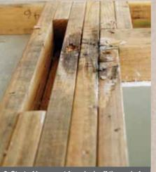
2. Start of brown rot from leak off the end of a head flashing
